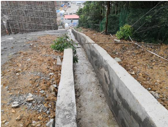
隧洞口截水沟
